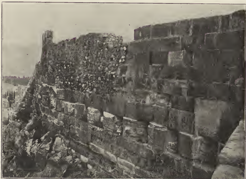
FIG. 23.—Drums of Columns of the Older Parthenon, built into North Wall.
